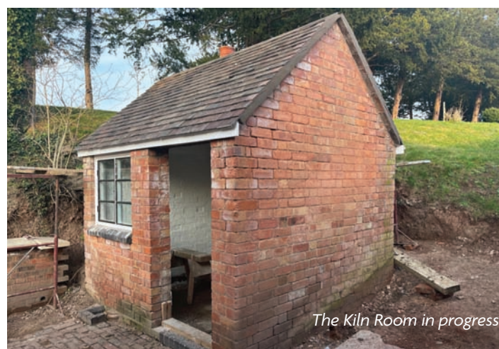
Constructing the Mosaic Garden
