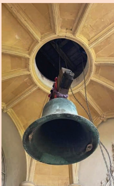
Bell being lowered through the hatchway
